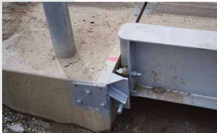
CAST-IN END ABUTMENT ANGLE
